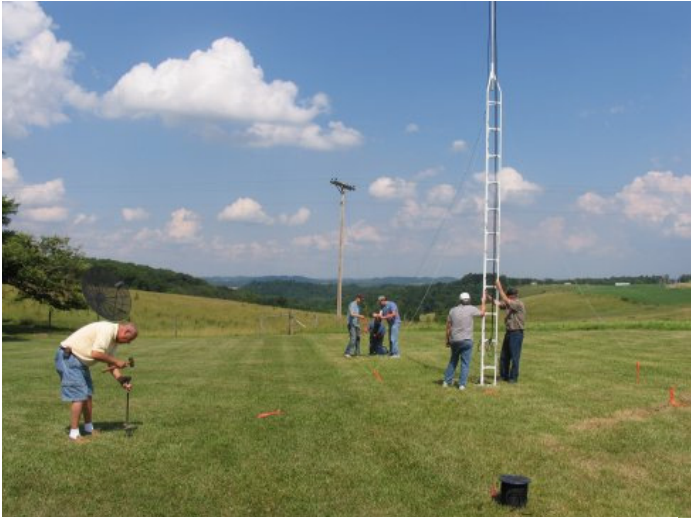
▲ Here are some of the guys setting up the tower and antennas for the event on Friday afternoon. {KL7RF photo}
